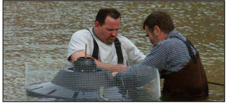
**Richard Wachel, left, and John Maxwell are waist-deep in the Reservoir Park Pond Apr. 2, hauling plastic bags, leaves and other debris that had clogged the spray fountain. After clearing the blockages, the installed a circular screen around the fountain intake, hopefully preventing a recurrence.**
